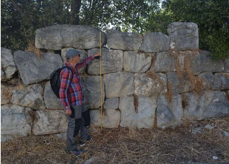
Fig. 4 Well-preserved wall-section built of hard limestone in polygonal masonry style. South of Myndos gate (P. Pedersen)
