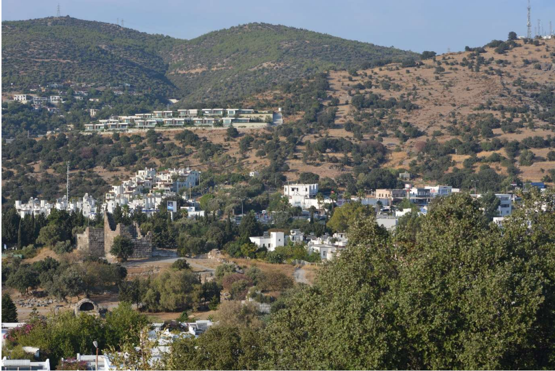
Fig. 2. Trace of the wall from the Myndos gate to the top of the Göktepe Hill (P. Pedersen).
