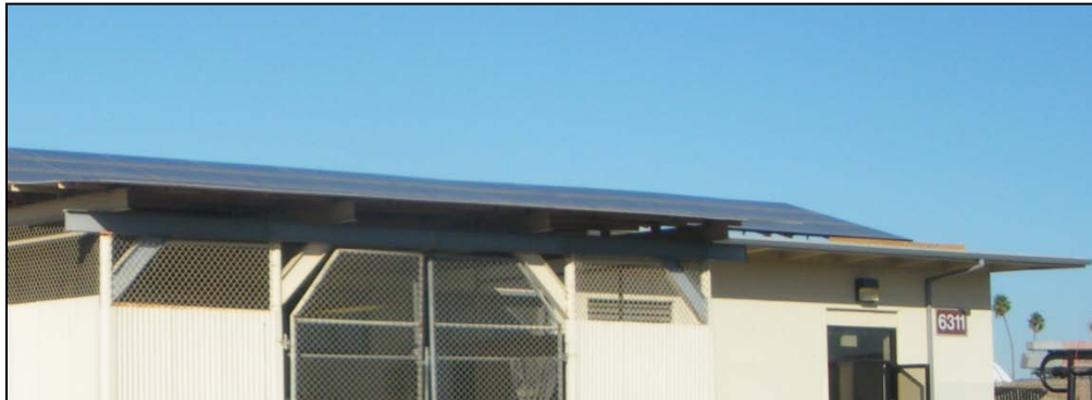
Figure 56. 30 kW PV System installed on building 6311 (Credit: Samuel Booth, NREL)
