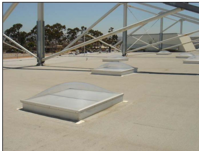
Figure 27. Daylighting system on hangar (Credit: NREL)
