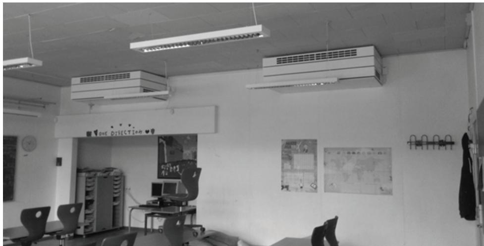
**Figure 5** New ventilation units installed in room 58.
