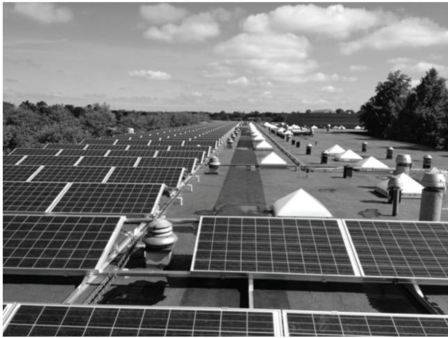
**Figure 3** PV installation at Stengårdsskolen: 220 kWp (209 Btu/s)—annual production 173 MWh (590 × 10<sup>6</sup> Btu).
