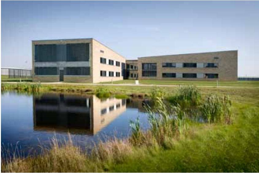
Ill. 3: The normal section seen from distance. Photo: Courtesy of Friis & Moltke.
