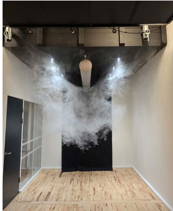
Ventilation test that shows how the ducts work.
