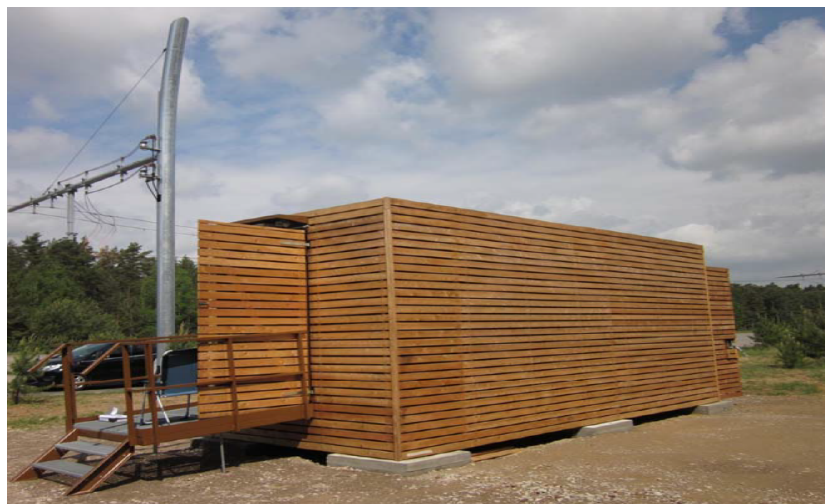
Figure 5.2: A traction substation [13]
