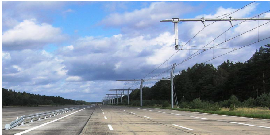
Figure 3.1: The setup of the Siemens eHighway. Vehicles connect to the overhead lines by using pantographs and receives electrical power [18].
