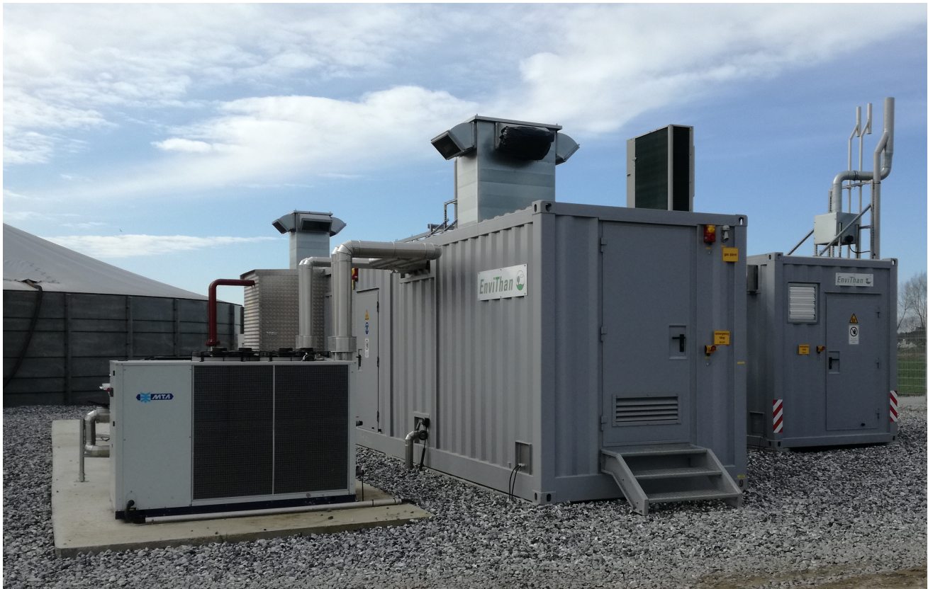
Figure 4.6.7: Membrane separation plant at Zastrow Bioenergi ApS
