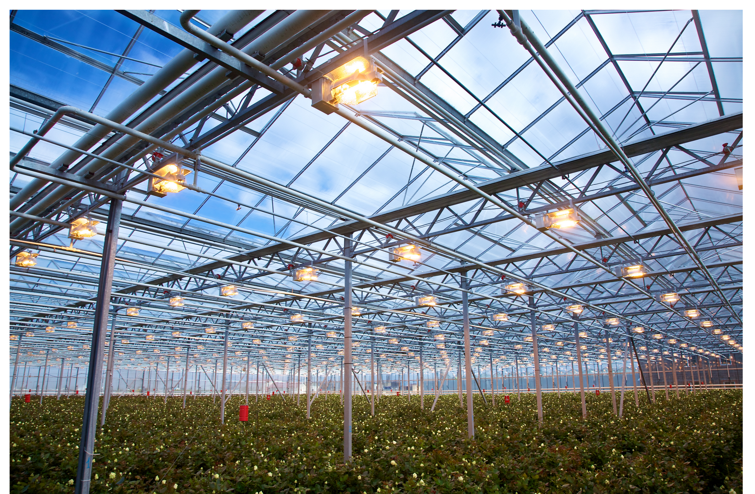
Figure 2 : Greenhouses is one of the many possible scenarios the project can be applied to.
