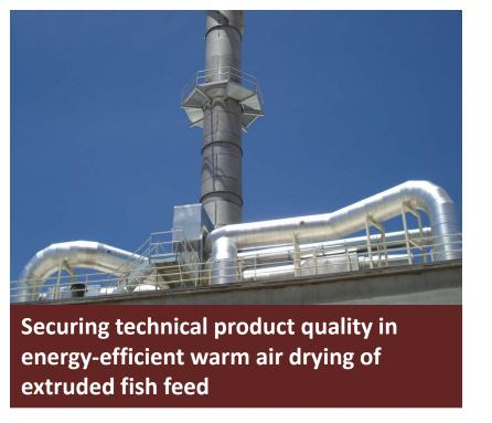
The drying of fish feed is a demanding process in terms of energy. In fact up to 65% of the total energy consumption in the production goes into drying. Graintec A/S is specializing in ecofriendly solutions, to which the new Ph.D. project is meant to contribute.
