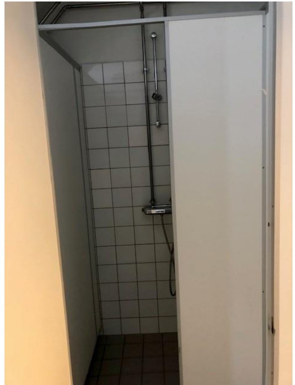
Shared bathroom (type A room)
