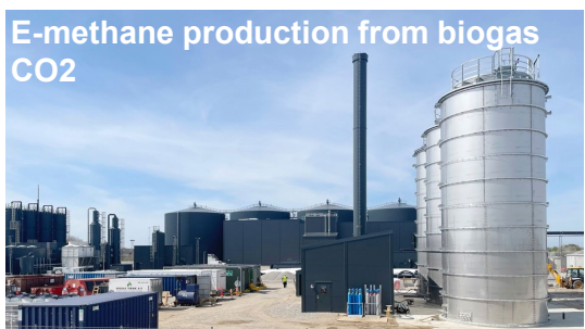
E-methane production from biogas CO2 Nature Energy, Biogasclean, Andel, SDU, DTU Glansager, near Sonderborg, Denmark Starting full scale (2023), 13 million m3/year (2024)
