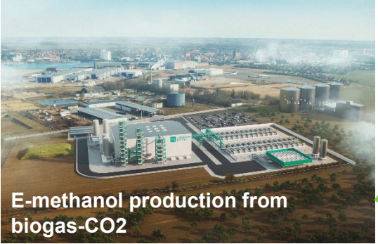
E-methanol production from biogas-CO2 European Energy, LEGO, Novo Kassø, near Aabenraa, Denmark 32.000 tons/year (2024) – to be used for POM plastic
