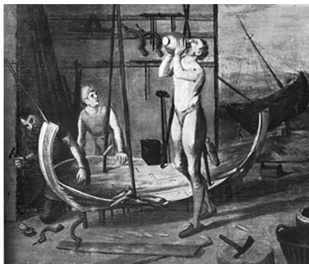
Figure 3-38: Dutch shipwrights building a clinker boat. Detail of a painting by a Master of Gouda 1565 (Friel, 1995 p.45)
