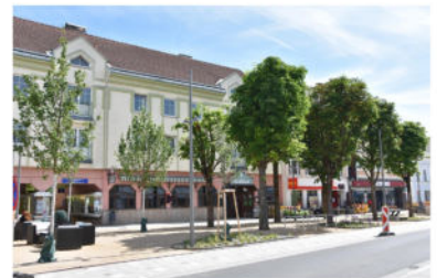
Europe's largest sponge city project in Amstetten © Stadt Amstetten
