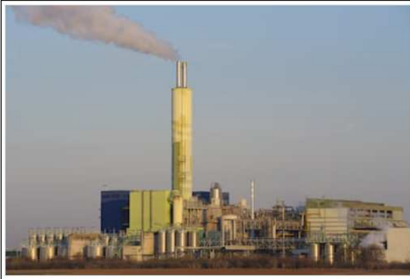
(Fig.37: Waste incinerating plant, Biebesheim, Hesse, Germany) 0
