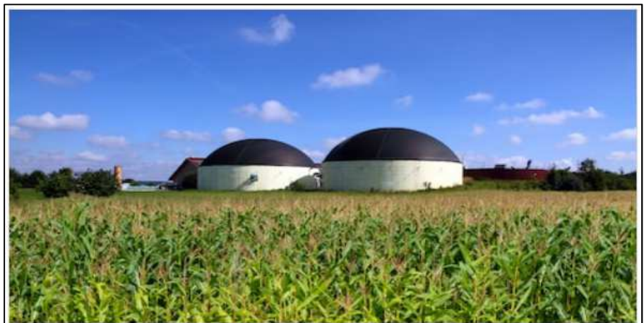
(Fig.36: Biogas production plant) 9
