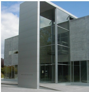
Building donated by The Møller Foundation
